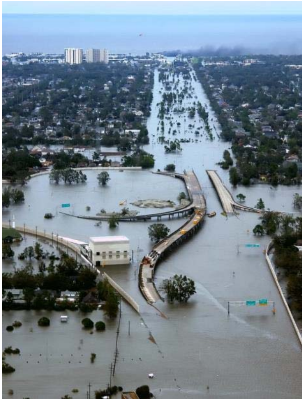
New Orleans after Hurricane Katrina, showing flooding at Interstate 10 at West End Boulevard, looking toward Lake Pontchartrain. (U.S. Coast Guard)
