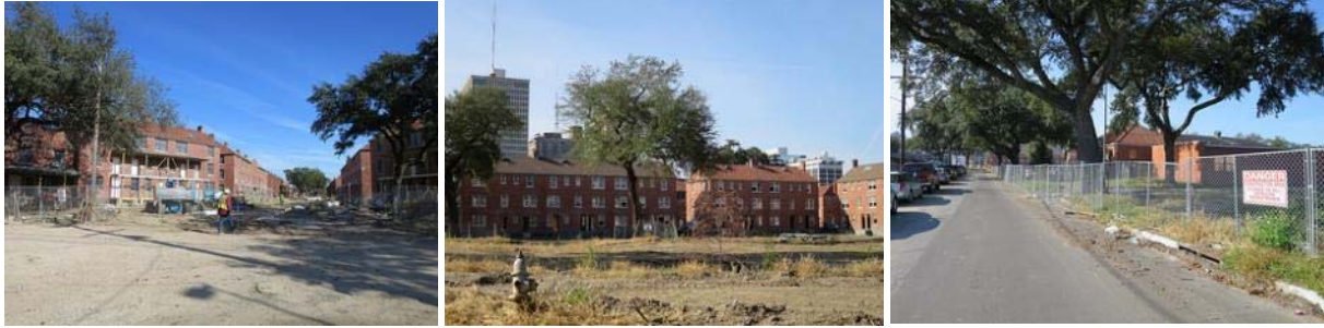
The new Iberville complex under construction.
