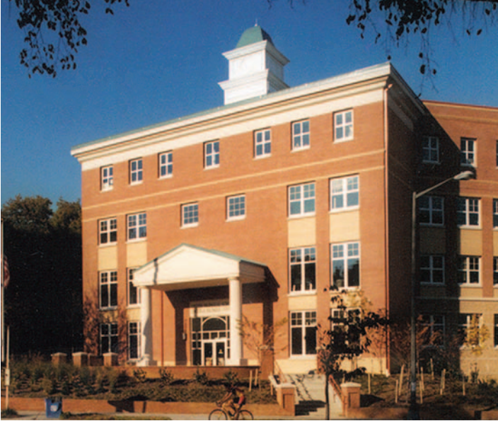
Contributing major benefits to the citizens of Washington, D.C., the James F. Oyster School/Henry Adams House, a public elementary school and 211-unit residential apartment complex, was constructed as a result of a partnership among the District of Columbia Public Schools, the community, and the developer LCOR Incorporated.
