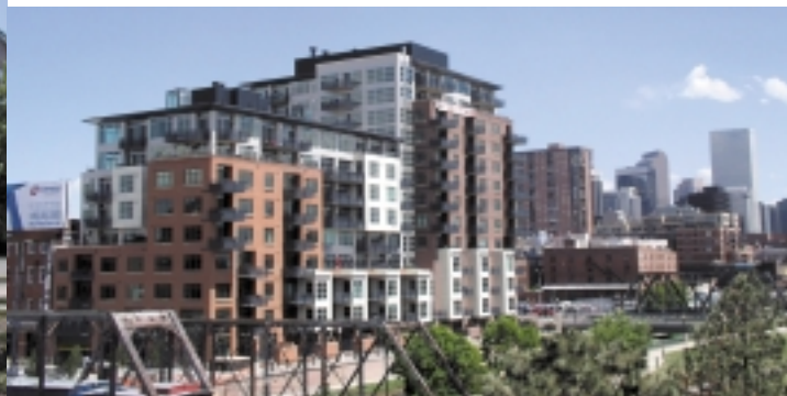
The Pepsi Center (left) and Waterside Lofts (below)—uses along the C Line.
