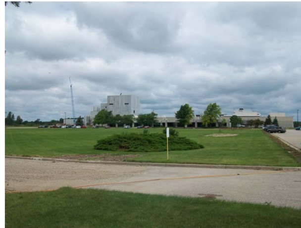
Building additions at the former Delphi Plant in Coopersville, MI
