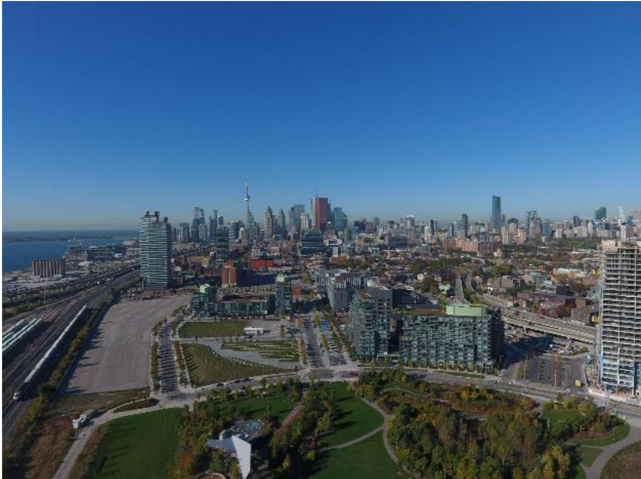
15. A view of West Don Lands from Corktown Common taken from the edge of the Don River. Corktown Common is positioned atop a flood-protection land form that protects 519 acres (210 ha) of downtown Toronto and unlocks the area's development potential. (Real Drone/ULI)
