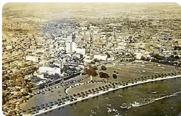
Stacy Park prior to the construction of NJ-29 (Source: The Trentonian )
