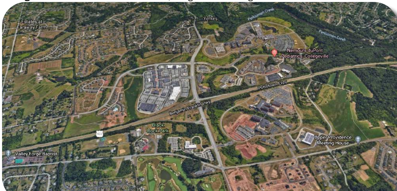
Figure 131 US 422 and PA Route 29, Image Source: Google Earth
