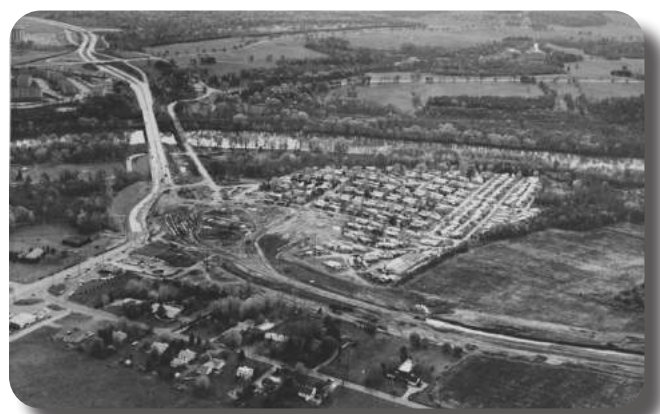
Figure 126 US 422 under construction at Valley Forge and Betzwood Bridge. Source: Temple Urban Archives
