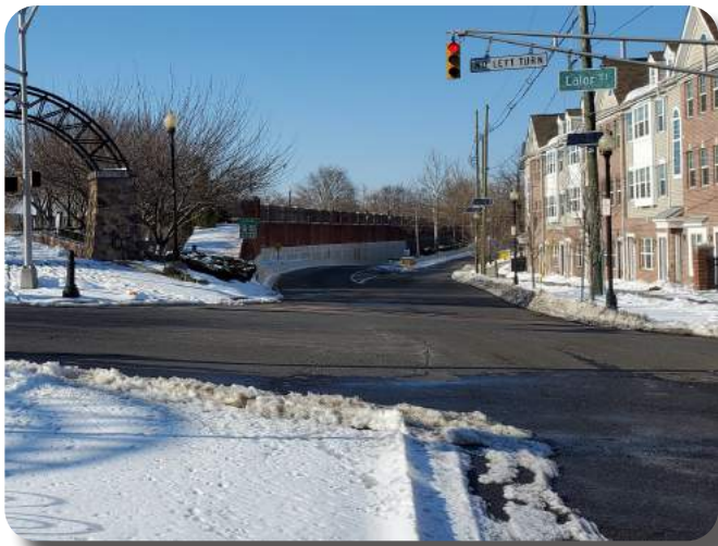
Figure 15 Entrance to the Lambertson Tunnel
