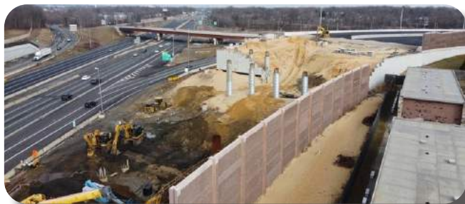
Figure 93 Direct Connection under construction, Source: 42 Freeway
