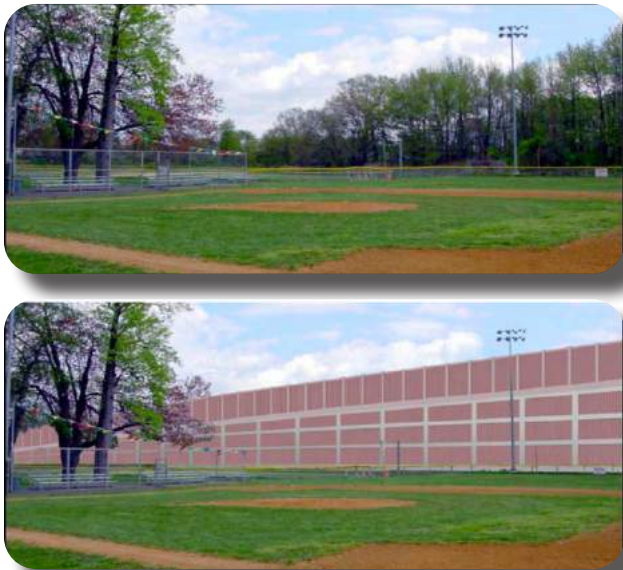
Figure 88 Bellmawr Baseball League field before (top) and after (bottom) construction. Source: EIS
