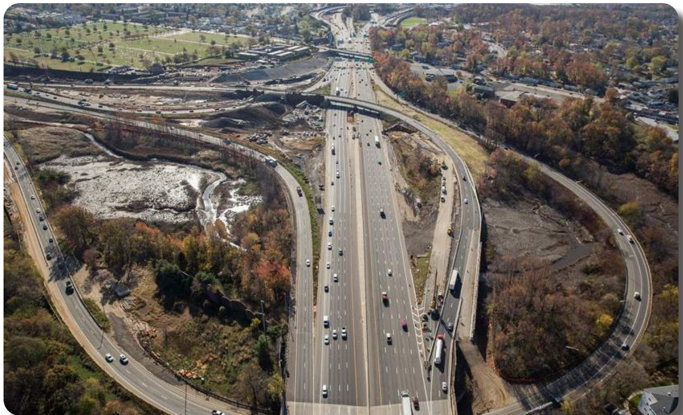
Figure 79 I-295/I-76/Route 42 Before Construction. Source: Stokes Creative Group
