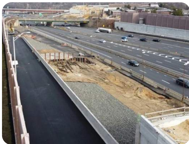
Figure 82 Direct Connection Under Construction. Source: 42 Freeway
