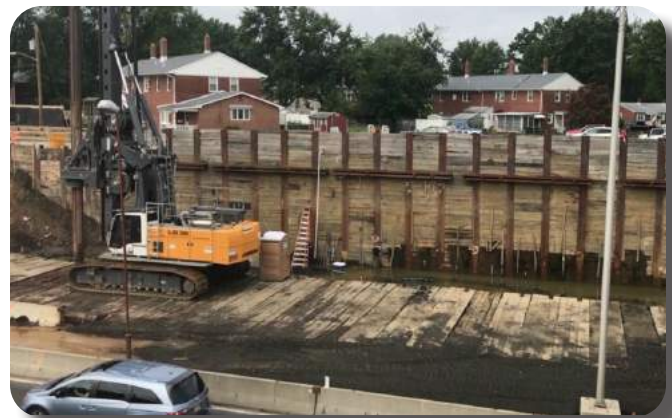
Figure 89 Residential impacts during Direct Connection Construction. Source: 42 Freeway
