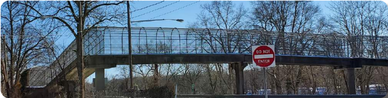
Figure 17 Pedestrian overpass over NJ-29
