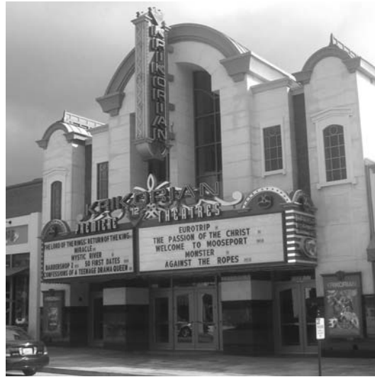
The 12-screen Krikorian Theatre, fronting onto Myrtle Avenue in Old Town Monrovia, has the look of a neighborhood theater, but a modern 12-screen facility flourishes in back. The theater has helped to make the Old Town scene lively.
