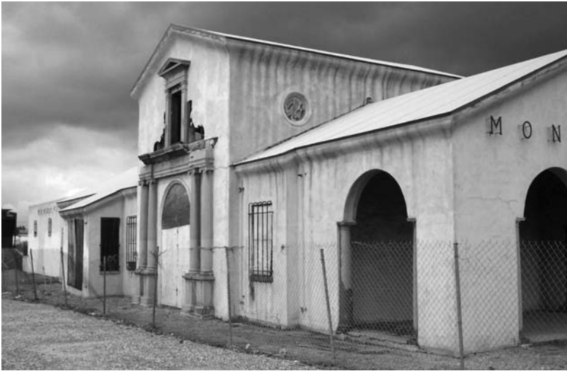
Above: Historic Monrovia Station on the Santa Fe Railroad will be restored and modernized to become the Monrovia Station on the expanded MTA Gold Line. Above right: Holly Street Village is a transit-oriented project in Pasadena near the end of the MTA Gold Line. The next phase of expansion of the Gold Line will extend to Monrovia and beyond.
