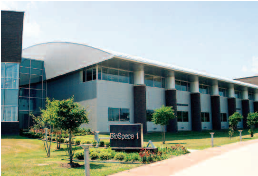
BioSpace 1, part of the Intertech Office Park.
