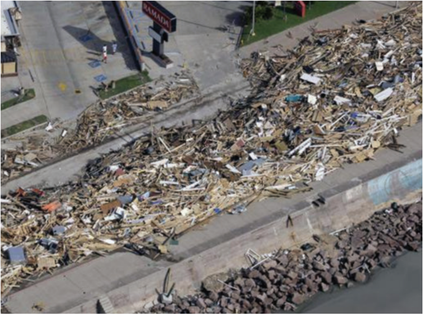
The seawall shortly after Hurricane Ike in September 2008. Ike ranks as the third most destructive hurricane to make landfall in the United States and is estimated to have caused over $3.5 billion in damage on the island.
