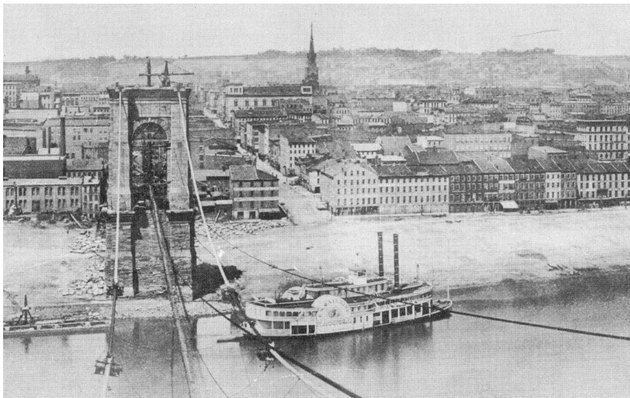
Figure 2. Construction of the Roebling Suspension Bridge, 1865. ( The Enquirer )
