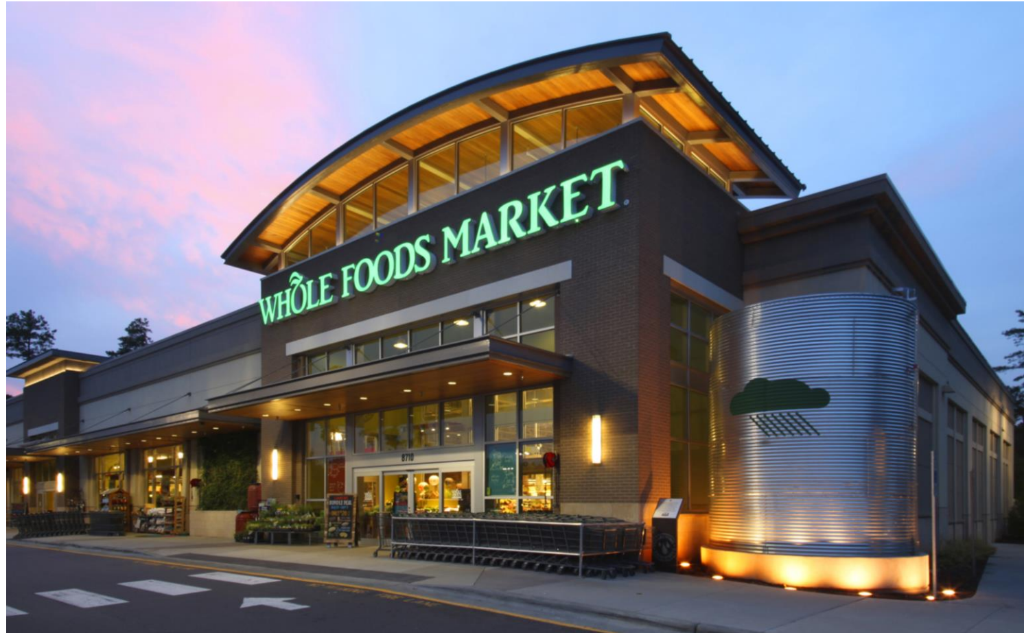
Market at Colonnade, photo courtesy Regency Centers
