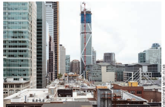
Construction of the Salesforce Tower above the Transbay Transit Center.
