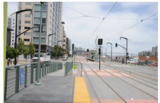
An at-grade railroad crossing at the Mission Bay site.
