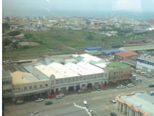
A view of the Sleeper site from the BCMM offices on Oxford Street.
