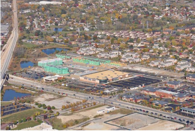
The center of the village of Orland Park: new living opportunities. VILLAGE OF ORLAND PARK
