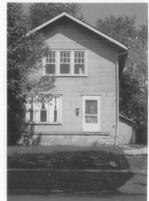
Figure 27. This residential building blends into its neighborhood even though all the windows have been covered over and the front steps are missing. The grounds are maintained and the special attention to decoratively protecting the window panels shows that the property is being well cared for until it can be rehabilitated. Photo: Ohio Historical Society.
