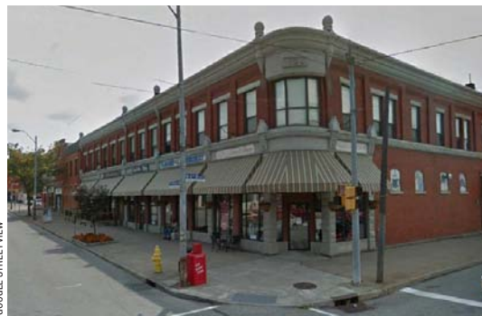
An existing mixed-use building along State Street.
