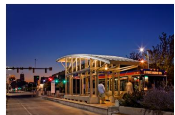
BRT station infrastructure in Kansas City, the Twin Cities, and Cleveland.
