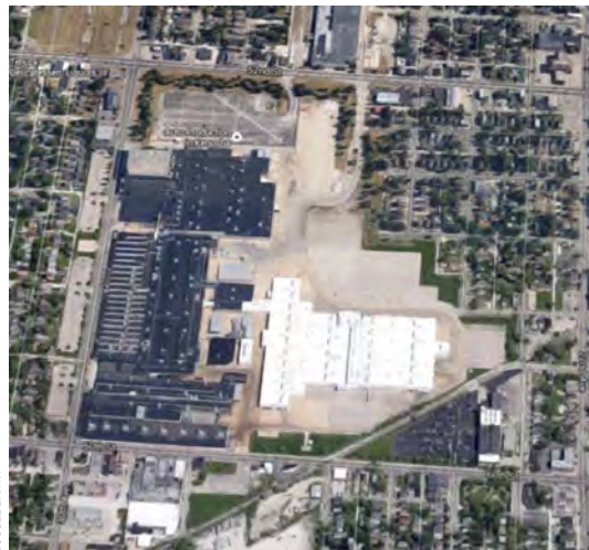
The structure of the Chrysler Engine Plant before its 2010 demolition.
