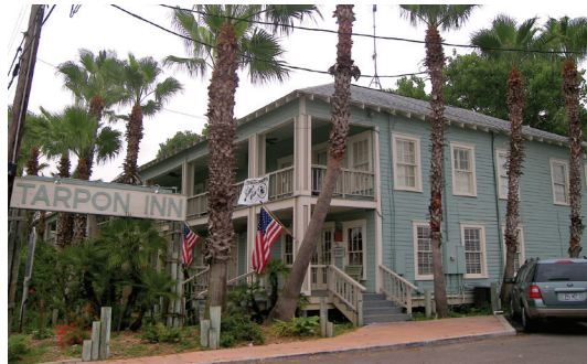
The historic Tarpon Inn, a well-known hotel located in downtown Port Aransas.
