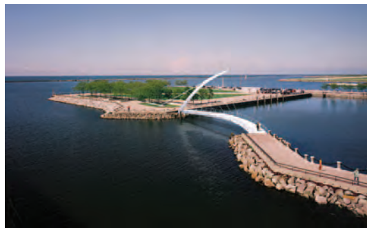
A movable bridge like the one pictured here can help better connect this area to the waterfront for active use by pedestrians and bicyclists.
