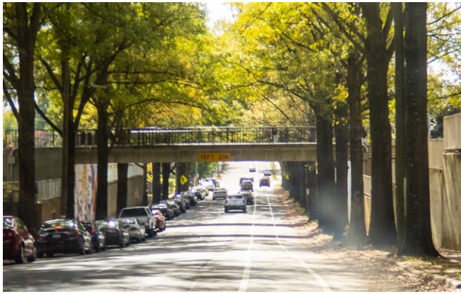
Currently, the Blount Street canyon's sole purpose is to serve as a thoroughfare for vehicular traffic. Redesigning this street could tap its potential and further extend the urban fabric of downtown and campus development.
