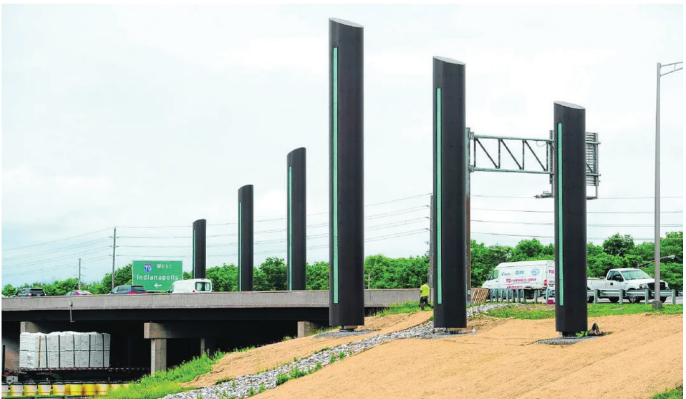
The gateway from I-70 into Greenfield is an example of the type of monumental treatment that will enhance the Mount Comfort Corridor.
