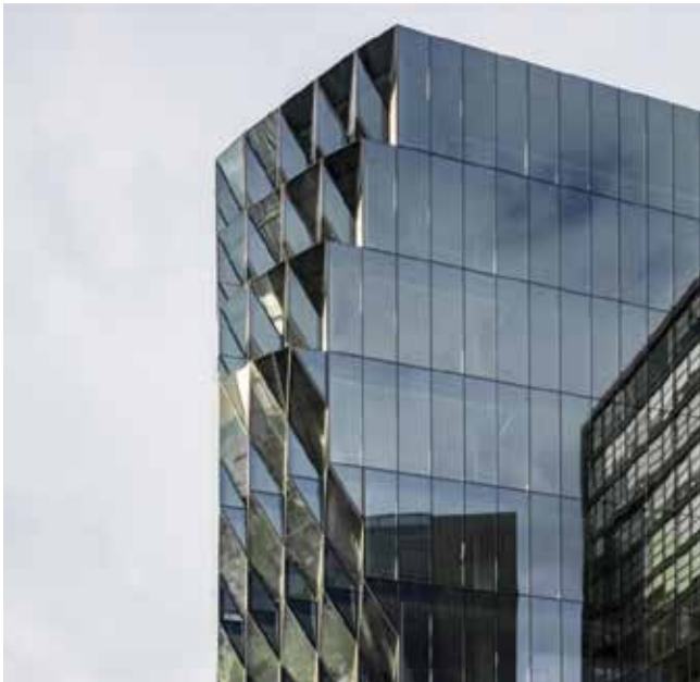
An example of solar carving by Studio Gang Architects at the High Line in New York City.
