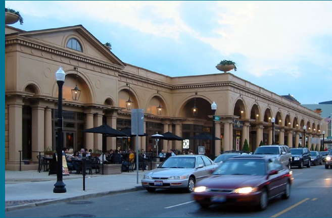
The Cap at Union Station in Columbus, Ohio, is an example of a stitch, enhancing North High Street as it crosses Interstate 670.
