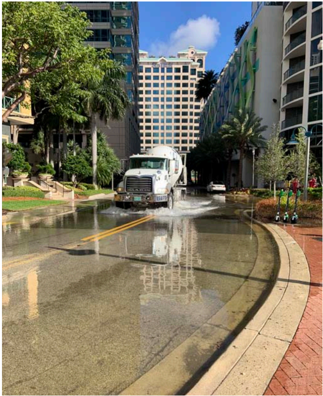
The panel observed sunny-day flooding, which is occurring more often as a result of sea-level change.
