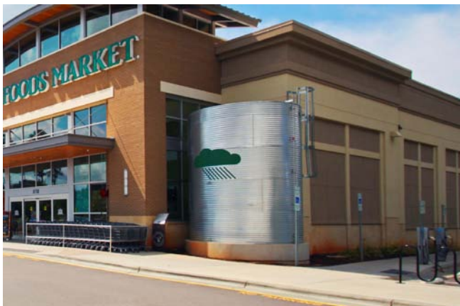
An above-ground cistern that benefits the development both as a marketing tool (symbol of Whole Foods' commitment to sustainability) and as a stormwater-harvesting vessel.
