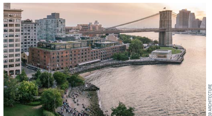
Empire Stores overlooks Brooklyn Bridge Park, which uses riprap edges to reduce the force of wave action.
