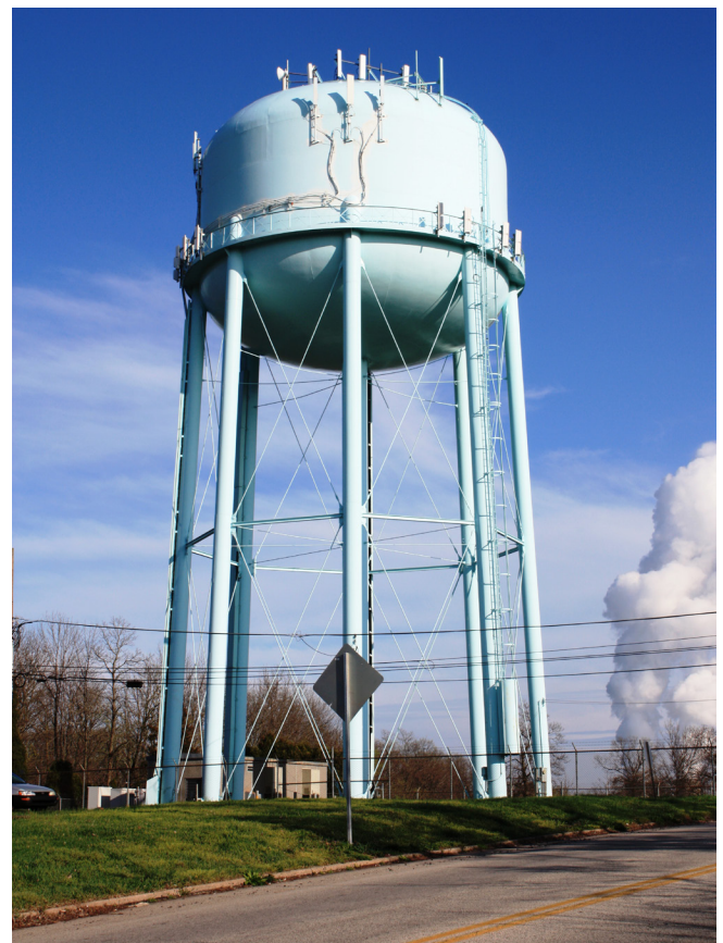
The Pottstown water tower can be seen throughout the borough and should be considered as a potential location for future place branding.
