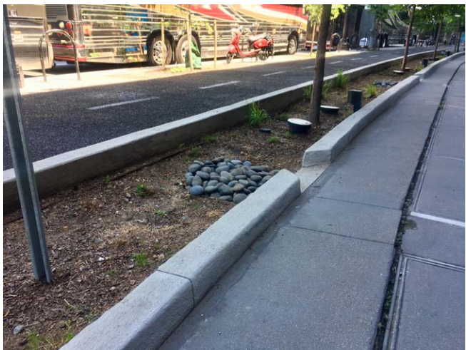
Curb cuts allow water to flow from impervious concrete on the sidewalk into a rain garden.
