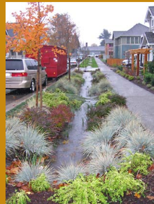
Bioretention swales, like this one at High Point, improve water quality, protect wildlife, and, most important, collect stormwater.
