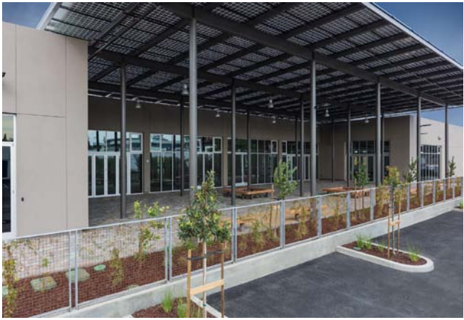
A net-zero energy building.
