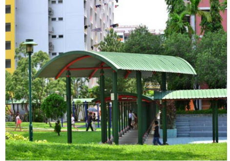
These pictures show how well Singapore maintains its old public housing estates, which were developed 40 to 50 years ago.
