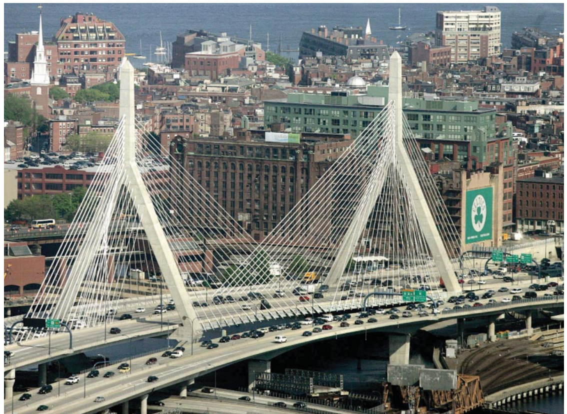
Boston's Big Dig is the nation's largest transportation infrastructure improvement project.
